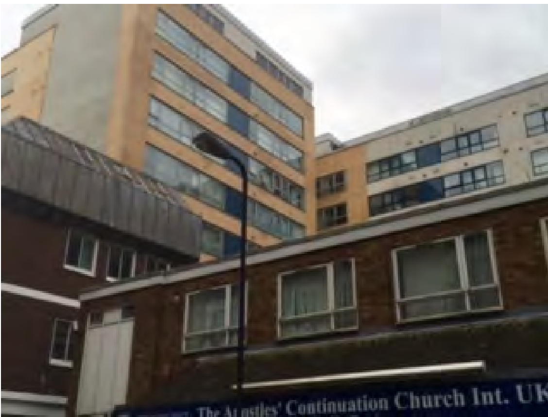
The rear elevation of the application site and Roxborough Heights
